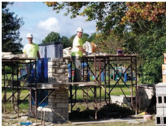
BAC Local 2 bricklayers Jason Dudek (right) and Chris Warfield (left) place the limestone, quarried in Lannon, Wisconsin, on the memorial's freestanding plaque.
