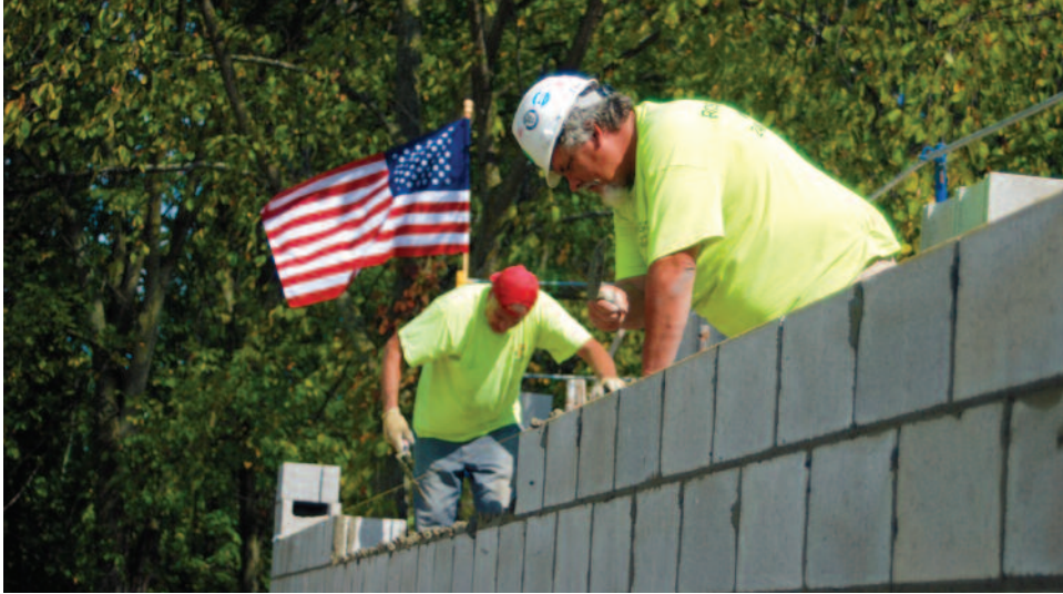
The American flag flies proudly as men from BAC Local 2 complete work on the memorial's CMU block core walls.
