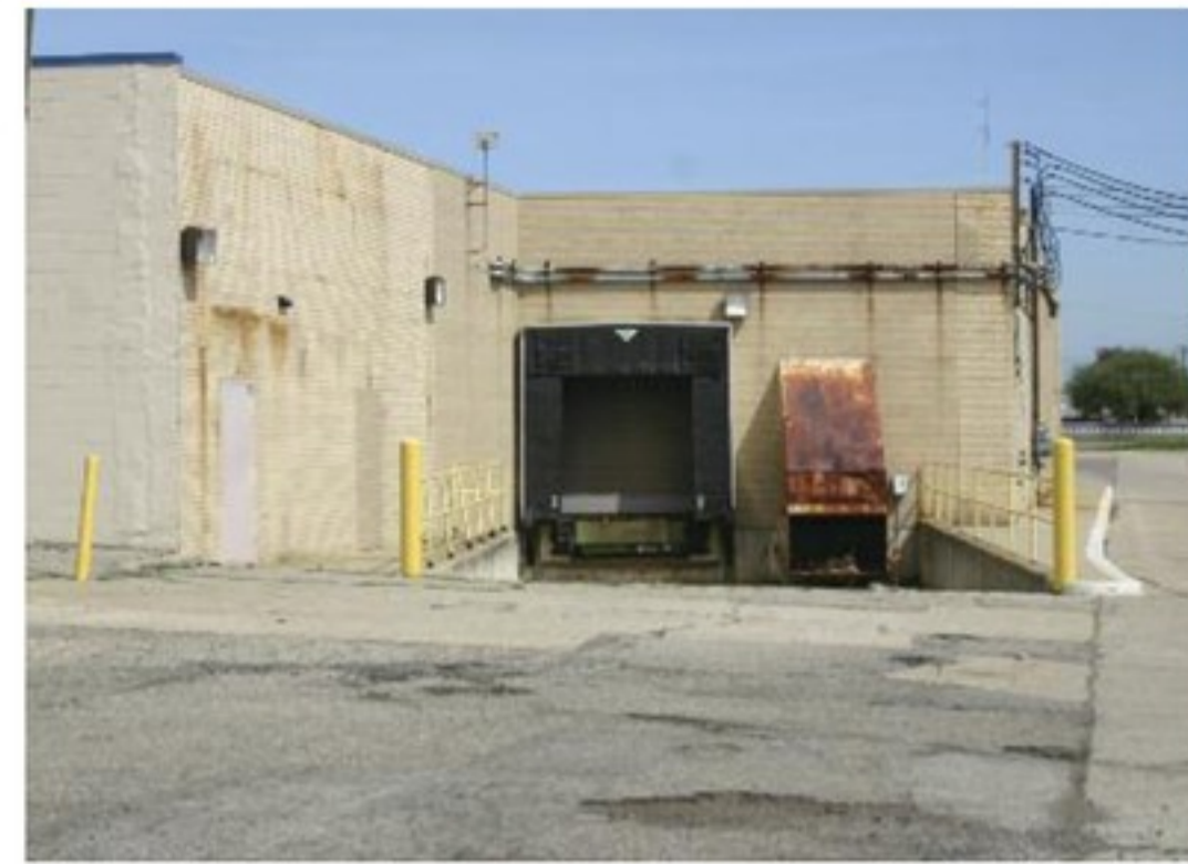
▲▲ Before and after views from 12 Mile Rd, of the old East Building – South Elevation.
